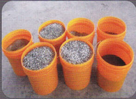
1. Prepare and weigh raw material (Cold Mix binder, quarry dust / sand & chip stones)
