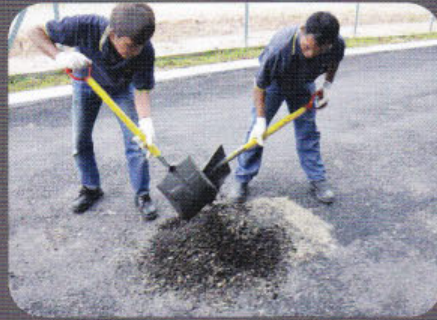
2. Pour Cold Mix binder into quarry mix. Mix evenly before use
