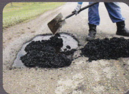
4. Pour the Cold Mix Asphalt into the target pothole then compaction
